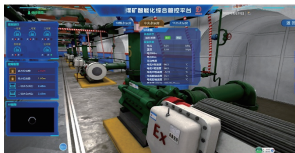
(b) 智能化煤矿 IGIS 水泵房工业管控应用 (b) Industrial control application of intelligent coal mine water pump house based on IGIS
